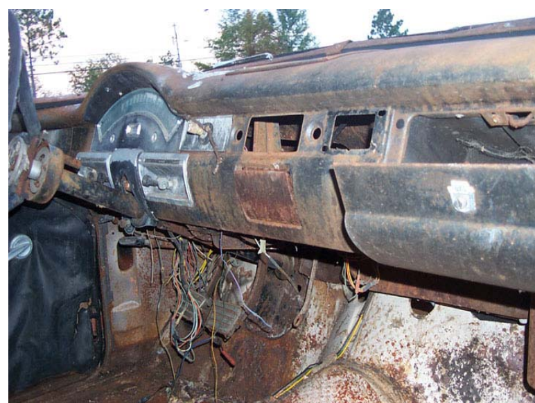
Most of the bad looking stuff is really superficial, surface rust. That makes it easy to get started.
